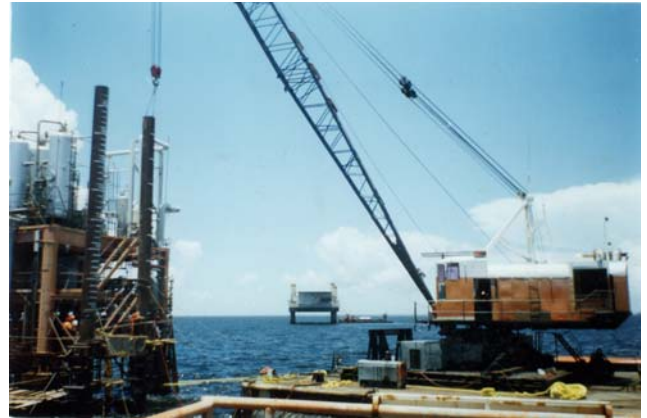
Piles being driven into the sea bed
