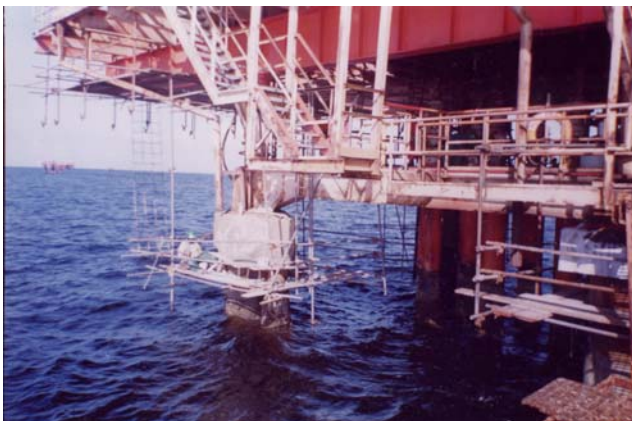
Pile-cap being repaired with HPRSTM™
