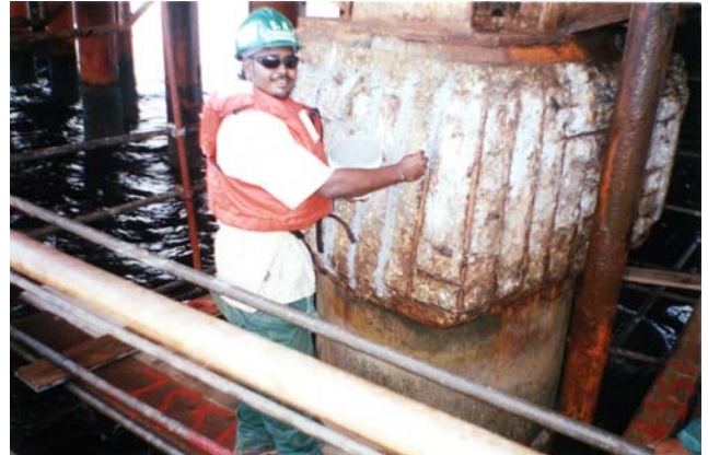
MCI®-2023 rebar coating applied on Pile-cap
